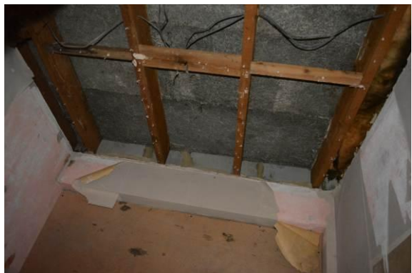
Figs. 11 & 12 Internal cavities beneath flat roofing
