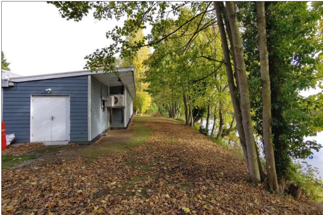
Plate 7: The mill pond and adjacent modern building
