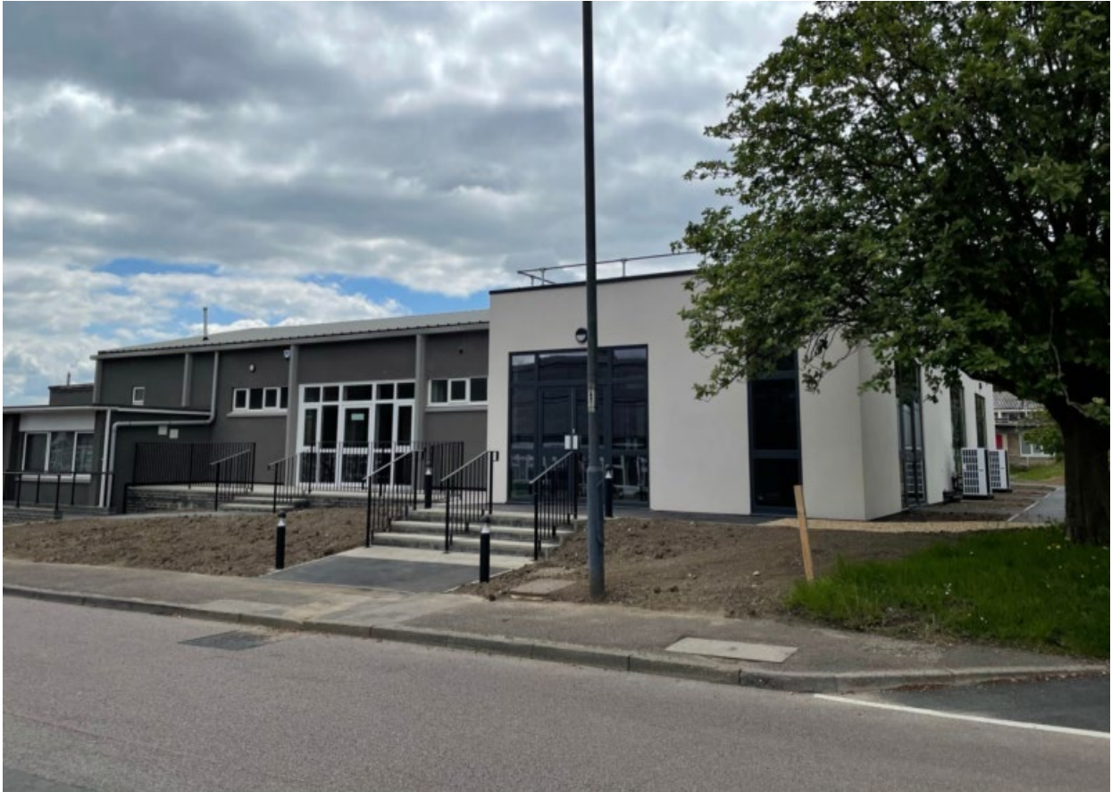
Figure 8 – Hollands Road Business Centre is a serviced office building which is managed by Suffolk CC. The building has recently been vacated by Menta and offers serviced space withing Class E. The building has also recently been refurbished. This is again a multi let building on short lease or tenancy arrangements and is therefore not comparable to the Boundary Road development.
