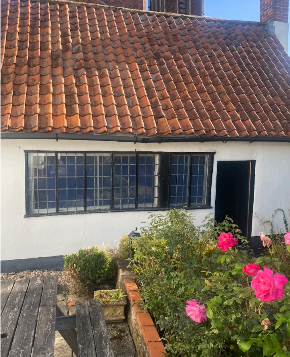
Building inc pathway - Site photo taken on the 13th of May 2026.
