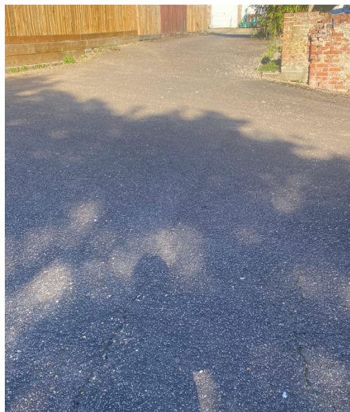
Driveway - Site photo taken on the 13th of May 2026.
