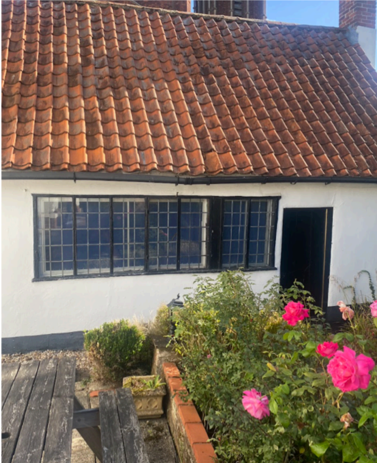
Building including pathway - Site photo taken on the 13th of May 2026.
