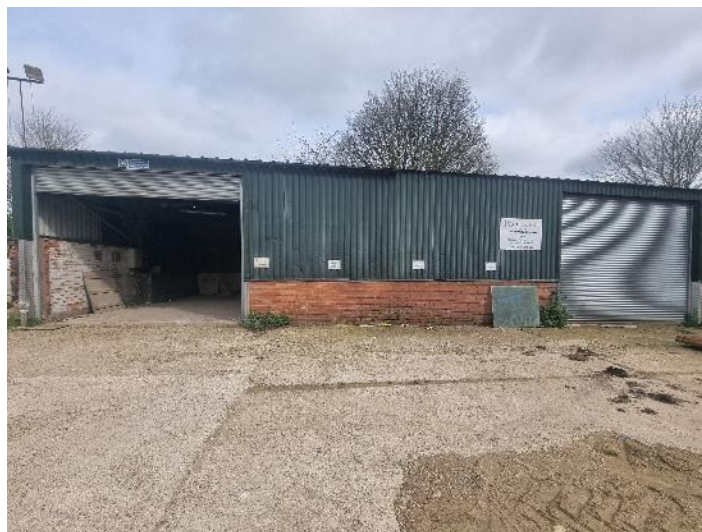
Figure 3: B1 in the eastern area of the Site.
