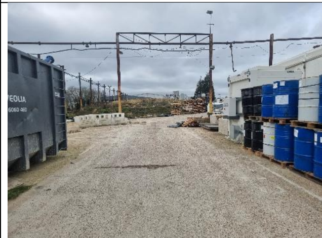
Photo 3: View of the Site from eastern aspect.
