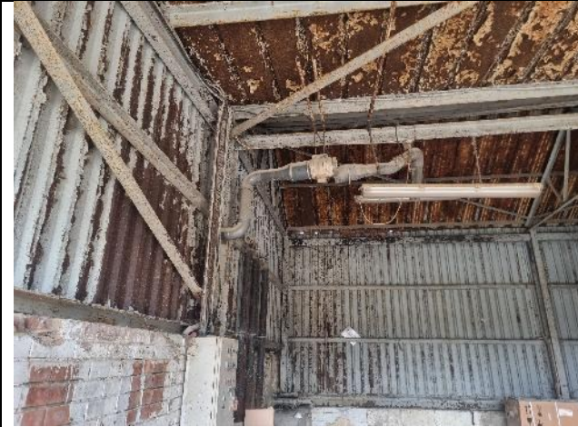
Photo 13: Internal view of the roof of B1.
