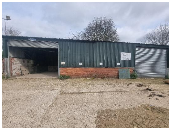
Figure 3: B1 in the eastern area of the Site.
