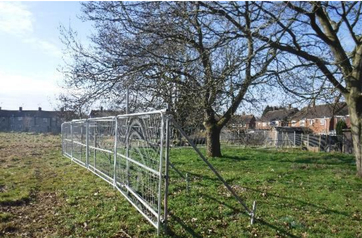
Figure 3: BS5837:2012 Examples of above-ground stabilising systems
