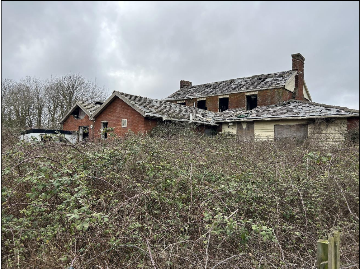
Plate 5 – Eastern elevation of the structure
