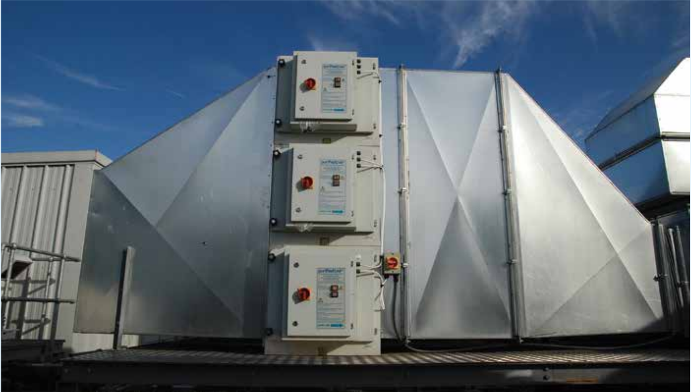
3 ESP Units Stacked in modular formation
