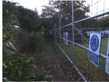
Figure 2: Alternative tree protection barrier example as recommended by BS5837:2012
