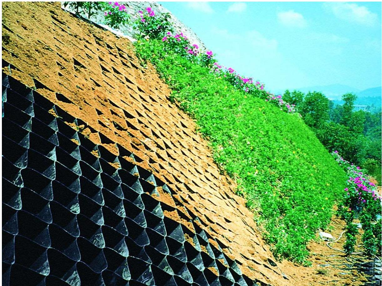
This system provides stabilisation to the existing earth bank without major structural works affecting the existing trees to Greenfields Way.
