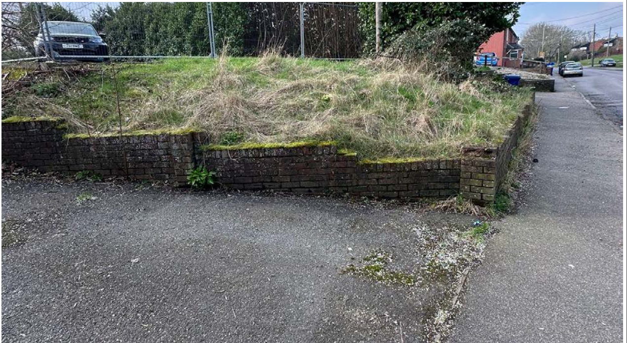
Photo 2: Grassed embankment with a small retaining wall along the access driveway in north of the Site.
