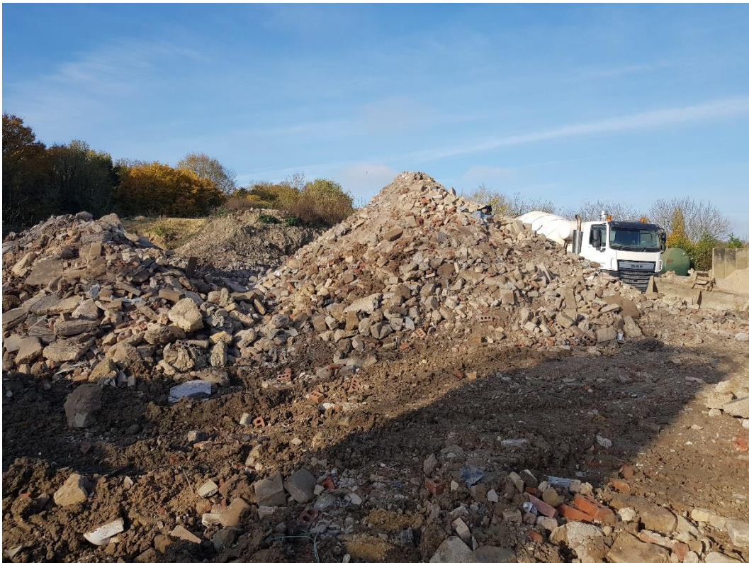
Figure 1.1: Construction and demolition waste being processed on-site (image source: DustScanAQ, 13/11/2024)
