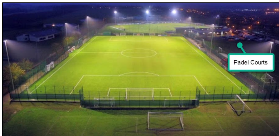
Figure 1: Aerial Photograph of the southern part of the Sports Complex, and Intended Padel Court Location
