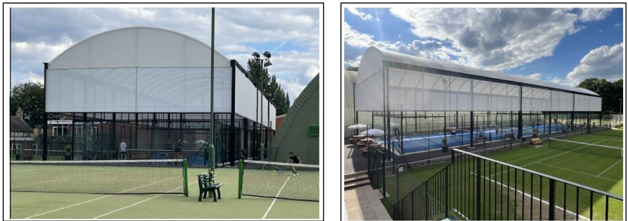
Figure 2: Photograph of Example Canopy
