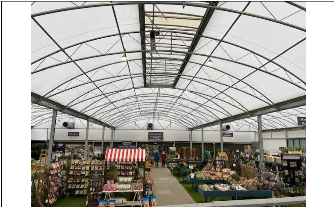
Photo 5 - White membrane roofs to Holt Garden Centre
