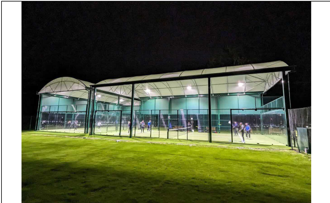
Photo 3 – Example of Green side panels and white membrane roofs showing no light spill above
