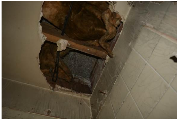
Figs. 9 & 10 Internal cavities beneath flat roofing
