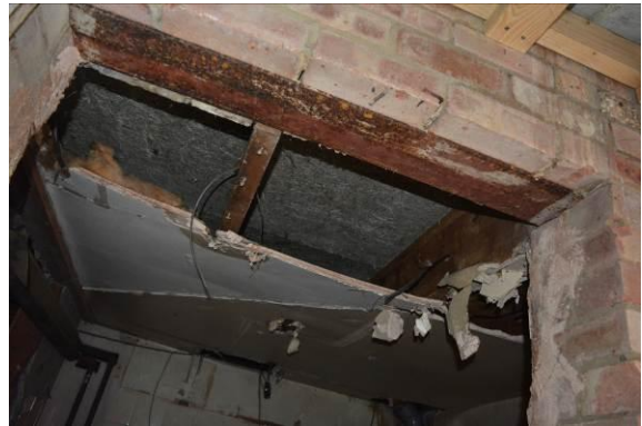
Figs. 9 & 10 Internal cavities beneath flat roofing
