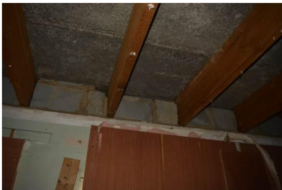
Figs. 11 & 12 Internal cavities beneath flat roofing
