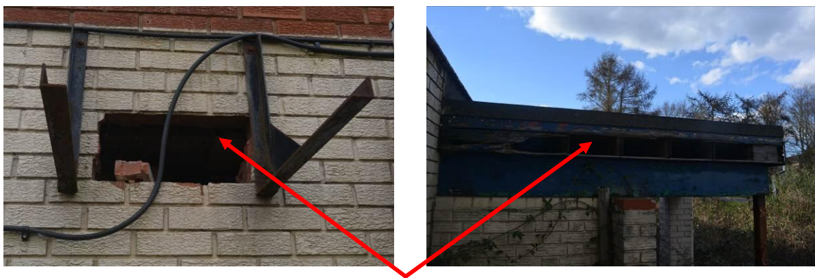
Figs. 5 & 6 External gaps and potential access points (arrowed)
