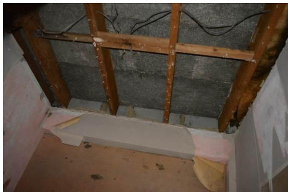
Figs. 11 & 12 Internal cavities beneath flat roofing
